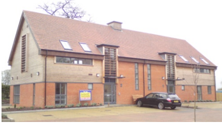
Units 1 and 2, Oakham Office Park
